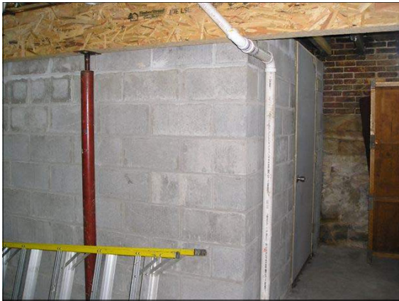
Construction in the basement
