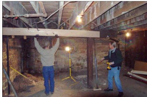
The floor in the back room kitchen area has a new support beam. The beam came as a gift from Montgomery Builders. Thank you JR for your "support". John Moon and his crew set it in place and added additional floor joist. Now this area of the building is secure.
